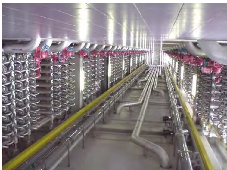
Photo 10. Example of Membrane Treatment Facility
