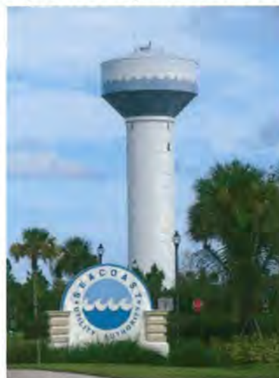
Photo 1: Seacoast Water Tower Hood Road Facility
