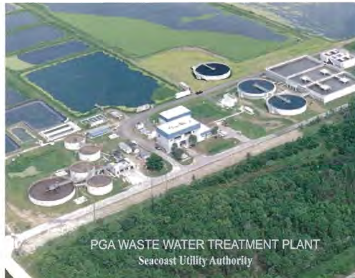
Photo 5: PGA Regional Reclamation Facility
