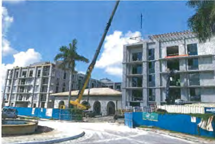
Photo 2. Construction progress photo of Solera at City Centre dated October 14, 2020.
